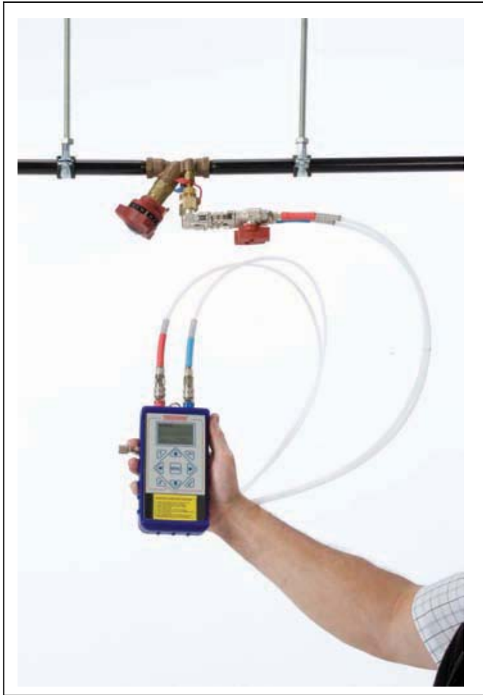
Figure 14: Digital differential pressure and flow rate instrument.
